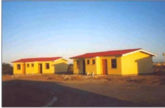
Figure 11 RDP houses sharing walls to save on construction costs and energy consumption. Source: (Jongeling 2001).
