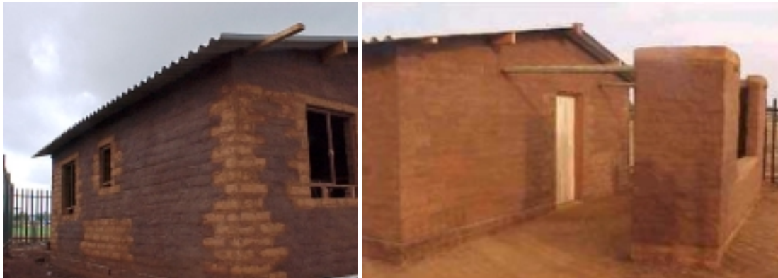
Figure 12 & 13 Midrand EcoCity mud brick house during construction
