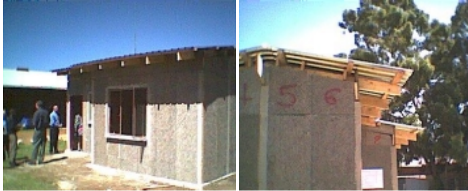
Figure 19 & 20 Innovative new materials for energy efficient houses in Benoni
