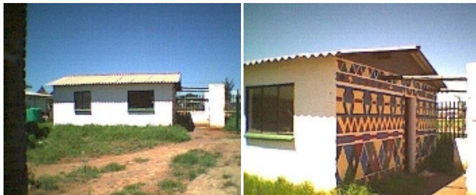
Figure 14 & 15 The mud brick house after completion and painting
