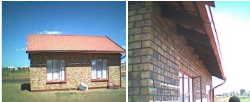
Figure 17 & 18 Brick house with cavity wall at Benoni
